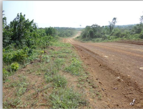
New Laterite Road (20km)
