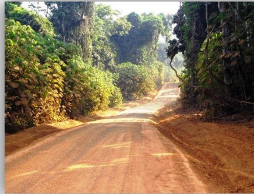
New Laterite Road (20km)
